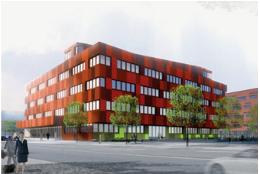
Der BioCube soll Ende 2012 fertiggestellt sein. The BioCube is due to be completed by the end of 2012.
